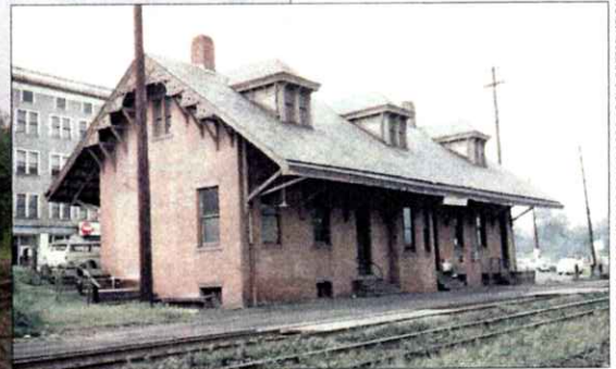
HISTORICAL PHOTOS COURTESY OF WINDSOR LOCKS PRESERVATION ASSOCIATION, INC.
